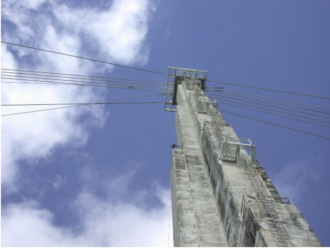
Figure 4.3 – View of Tower-Top, Mainstay and Backstay Cables.
